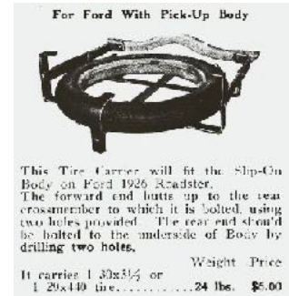
Above: Clymer Ad for an Underslung Tire Carrier. Below: View of the fabricated tire carrier from under the T. Below Left: View of tire carrier on the T. Ad scan and photos by Paul Duncan, September, 2024.
